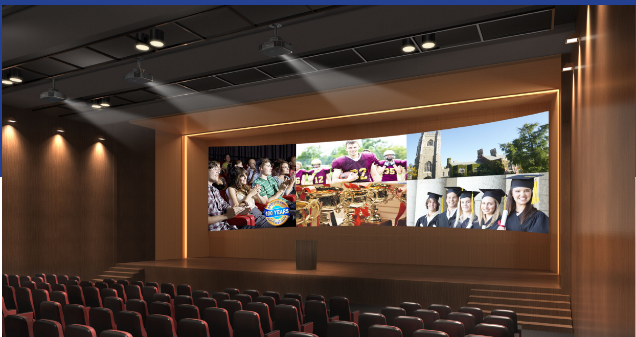
Multiple projectors used with a super-wide, curved screen — a simpler alternative to the dvLED equivalent. Disclaimer: Images have been simulated.
